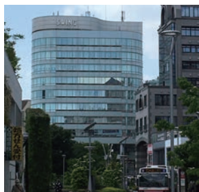
Musashino Swing Building
