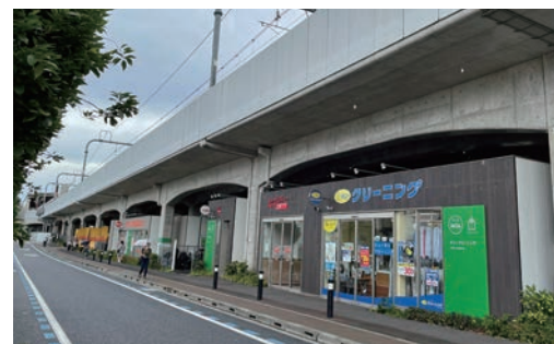
Connects the South and the North side of the station.
